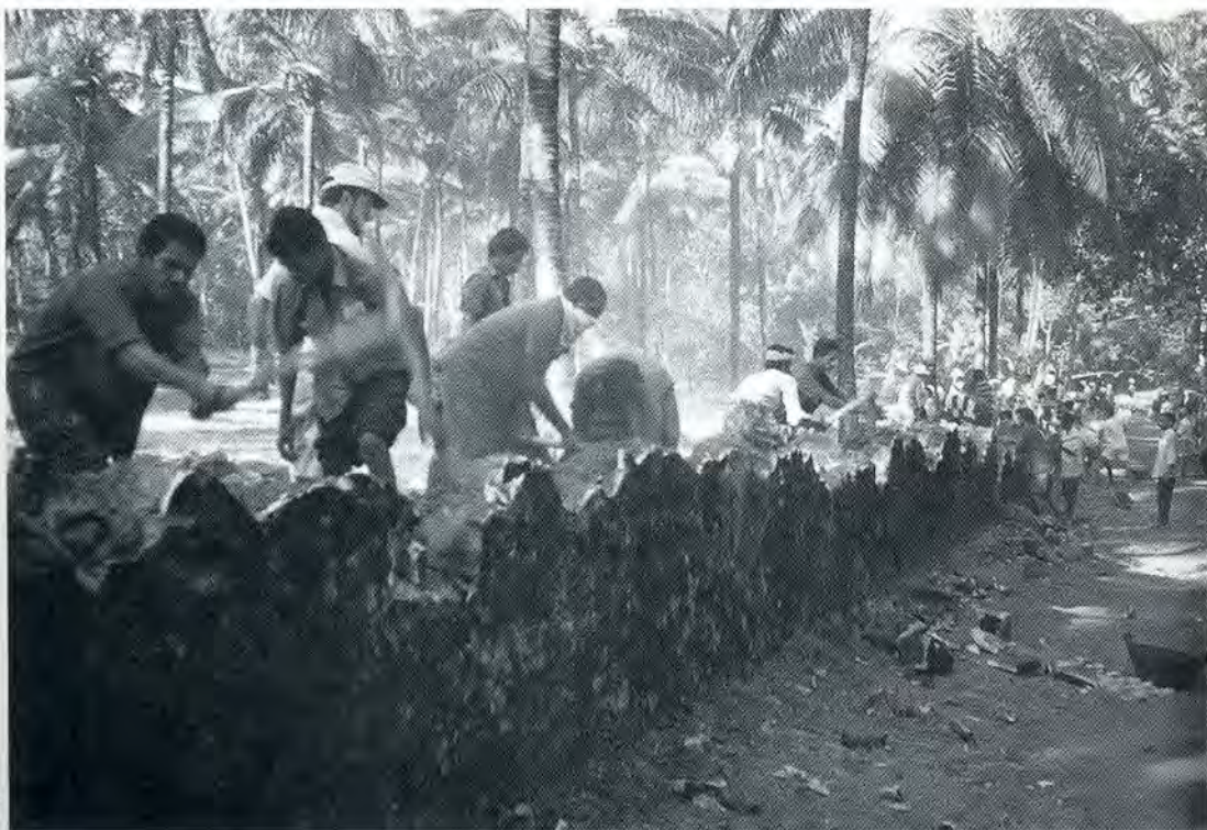
The work portion of RYS began with the goal of widening 1.2 km. of road.
